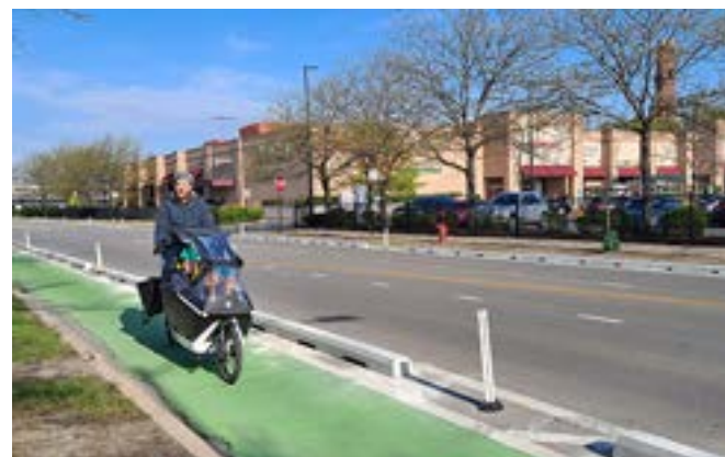
Prefabricated concrete curbs on Roscoe Avenue (CDOT)
